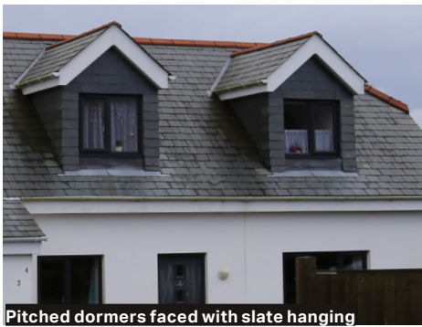
Pitched dormers faced with slate hinging
