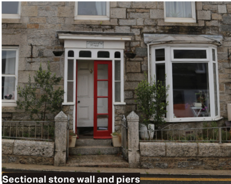
Sectional stone wall and piers
