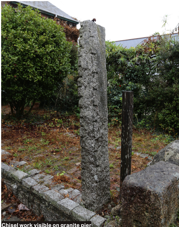
Chisel work visible on granite pier
