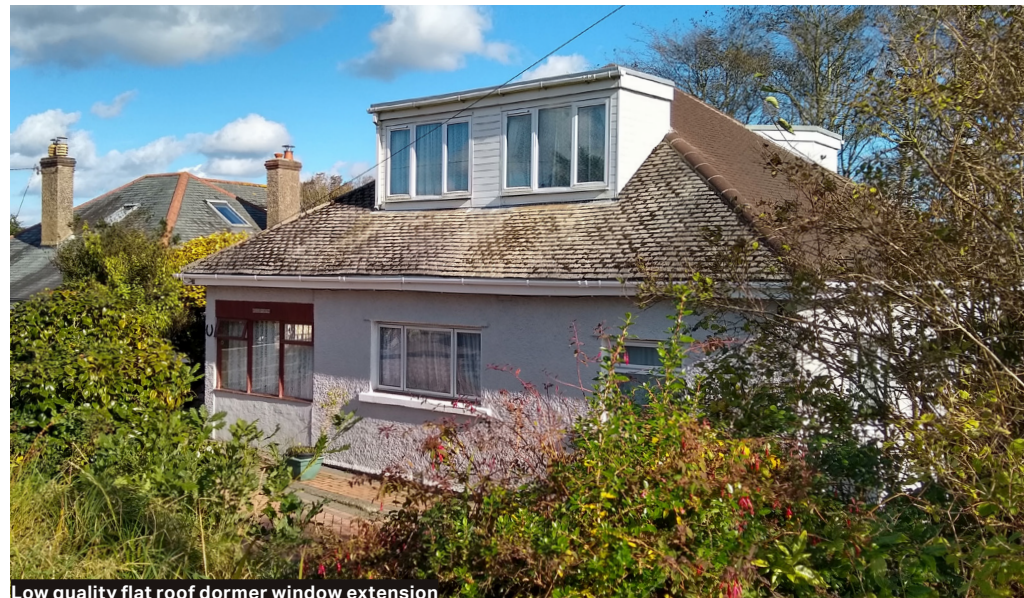
Low quality flat roof dormer window extension
