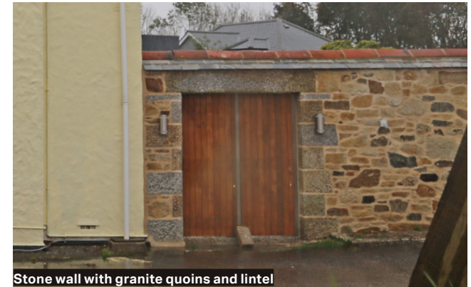
Stone wall with granite quoins and lintel
